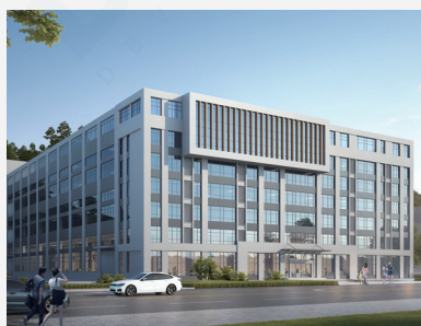
Company Headquarters (Under Construction)
