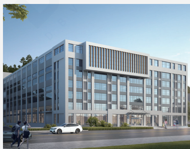
Company Headquarters (Under Construction)
