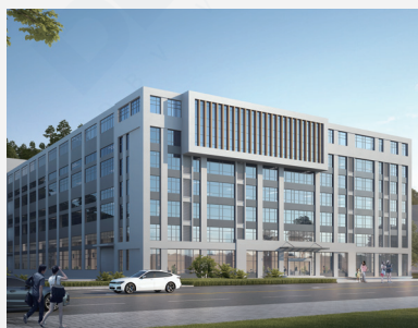
Company Headquarters (Under Construction)
